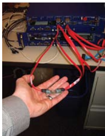
Figure 4: Test Setup to Avoid: Signals are 1) sent over a splice, 2) the extended double cable is longer than required, and 3) the cable used is unshielded.
